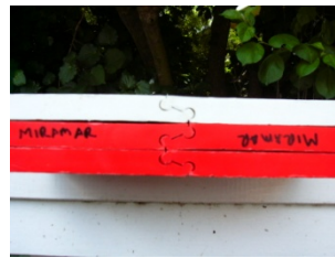
Incorrect(middle board facing wrong direction)
